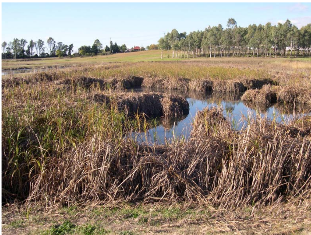
Figure 4. A FWS CW for tertiary treatment of municipal wastewater in McGrath Hill, Hawkesbury, near Sydney, NSW, Australia. Photograph taken by the author.
