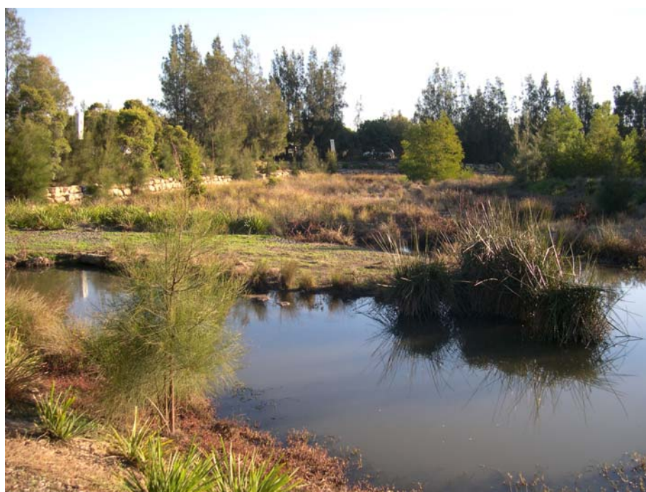
Figure 2. A free water surface constructed wetland (FWS CW) for stormwater runoff in Woodcroft Estate near Sydney, NWS, Australia. Photograph taken by the author.
